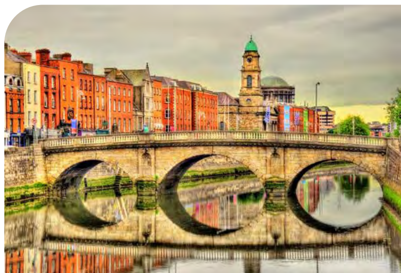
Mellows Bridge – Dublin, Ireland
